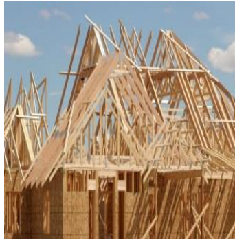
Building wooden skeleton Cost: $40,000
